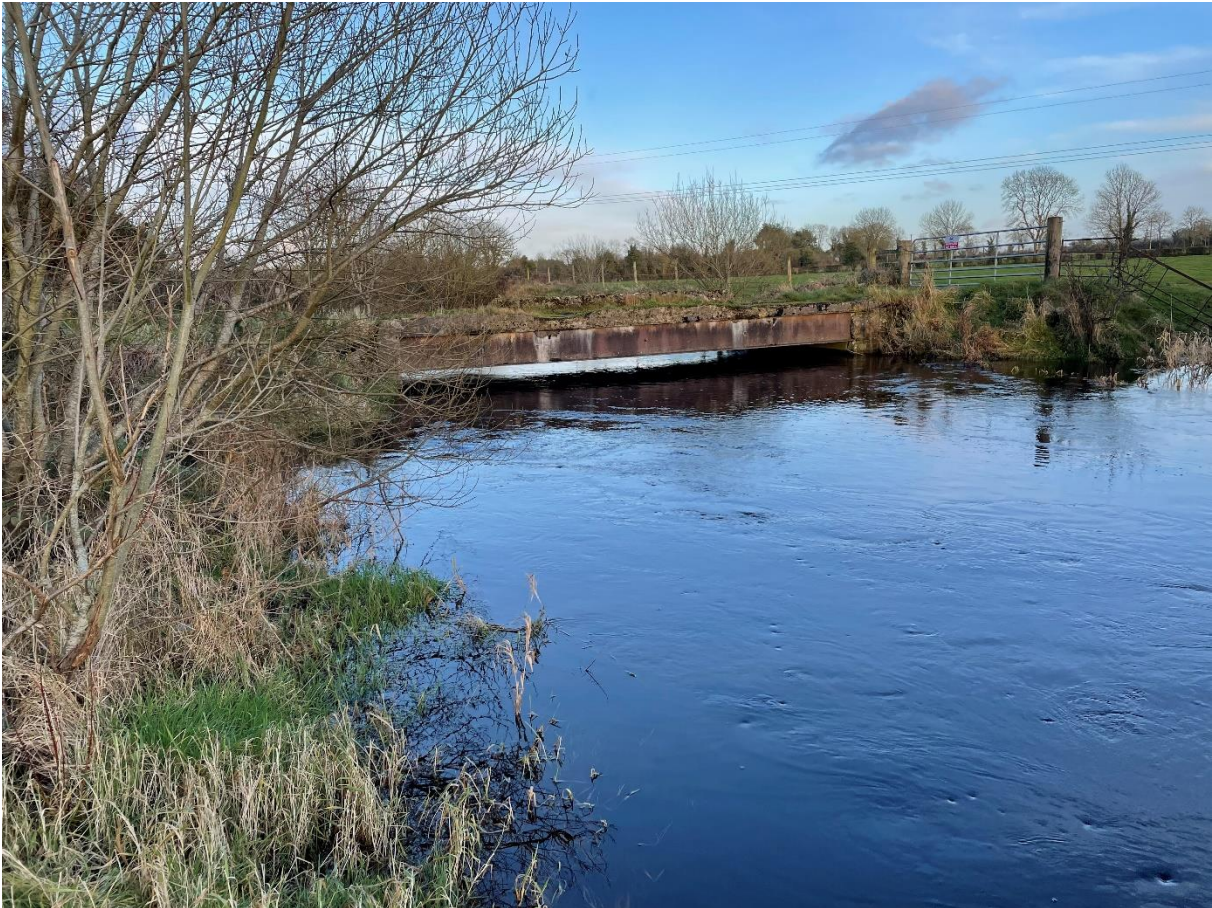
Photograph 2 - downstream bridge facing upstream
