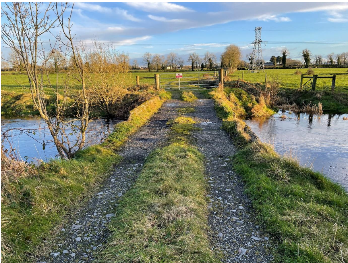
Photograph 1 - downstream bridge facing east
